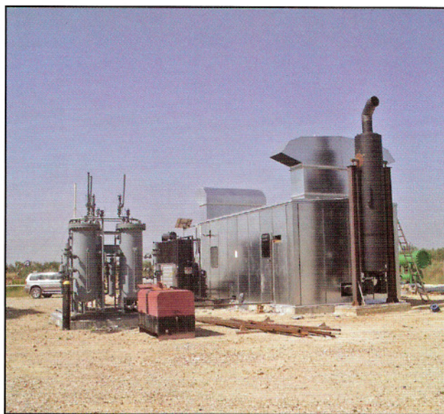
■ Two views of the completed compressor installation that will host the first Ajax integral compressor with CE marking. The site is in Spain's Guadalquivir Valley in Andalucía, not far from the city of Seville.
